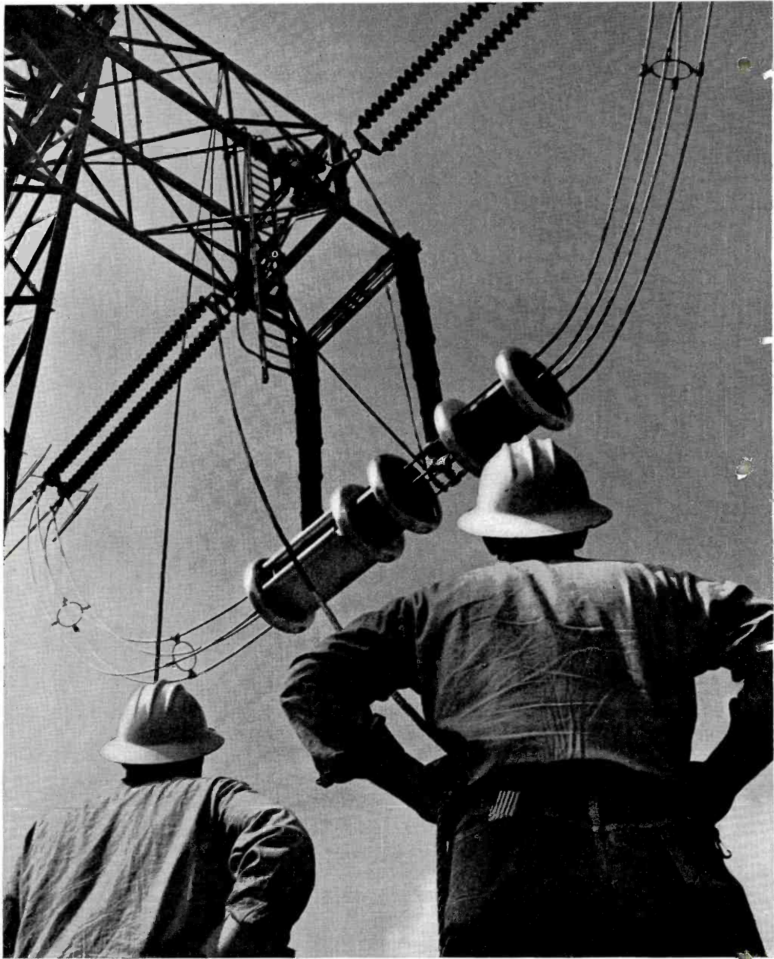
Extra-High-Voltage Transmission (EHV). As power needs grow in the future, electric lines will have to carry greater loads with greater efficiency. Under research conditions, an investor-owned power company and a manufacturer have achieved 775,000-volt transmission (most high-voltage lines today operate between 115,000 and 345,000 volts).
